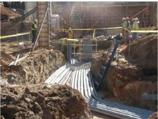
Figure 1 Underground utility building feeds.
